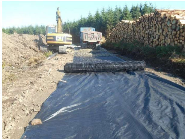
Figure 6: Crushed Rock Roadway & Crushed Rock Roadway Build-up with Geotextile
