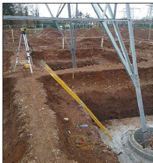
Figure 2: Stepped Back Excavation
